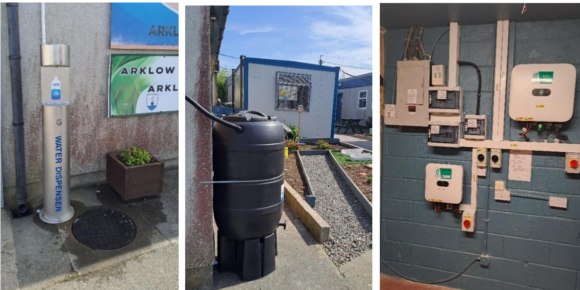
Arklow United FC, water refill, rainwater harvesting, inverter and smart switches for Solar PV installation
